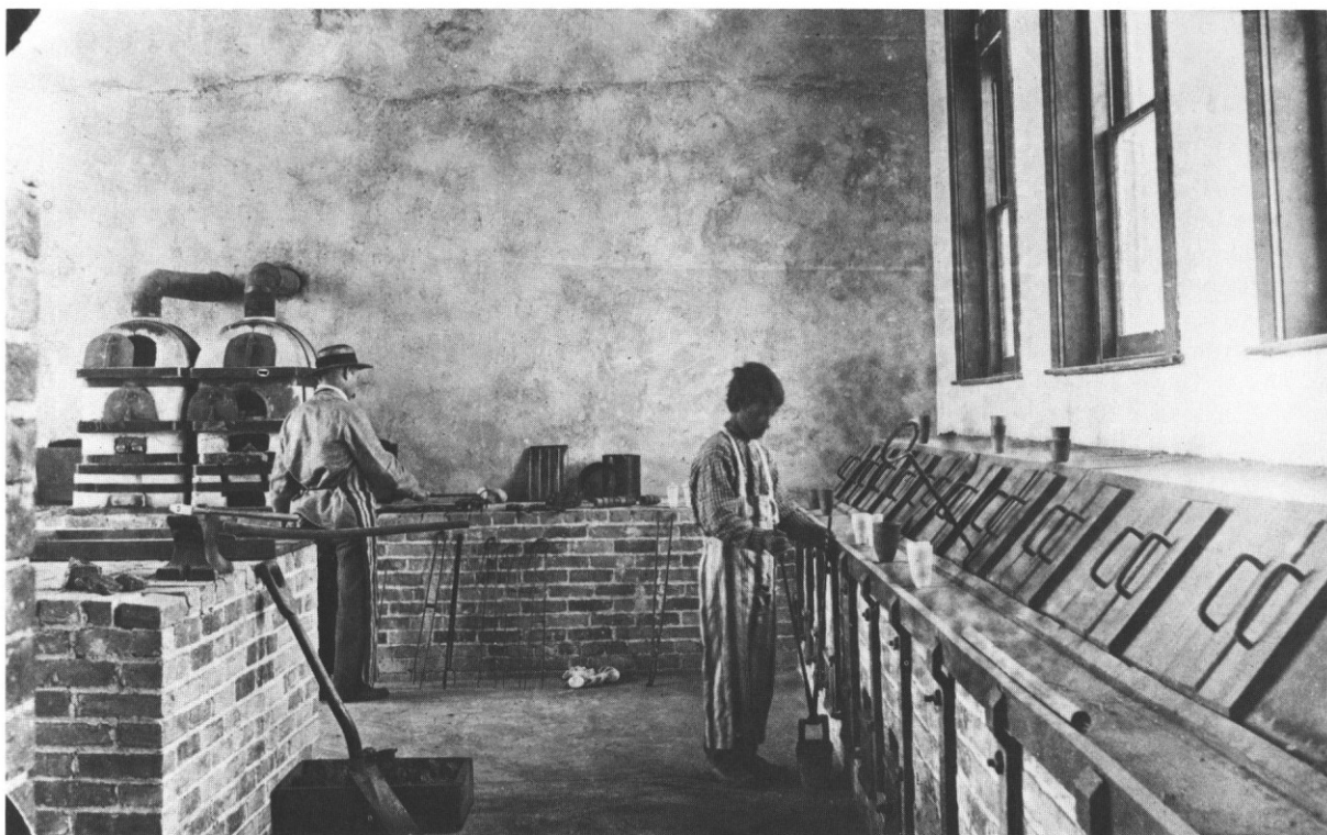
Assay lab and sampling department, Billing smelter, ca 1885. The plant metallurgist was all-important to the financial success of any smelting works: the reputation of the business rested in large part on his honesty and expertise, while ores were purchased and furnace charges made up on the basis of his analyses. Pictured here is doubtless Mr. Furman, "knight of the crucible and tongs" who would later become a prominent metallurgist in his own right, and his laboratory assistant. Photo by Joseph E. Smith, courtesy Ed Smith; New Mexico Bureau of Mines and Mineral Resources collection.
