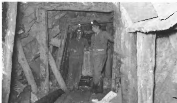
FIGURE 8. Drift on vein (1952). Ore stopped above and below level.
