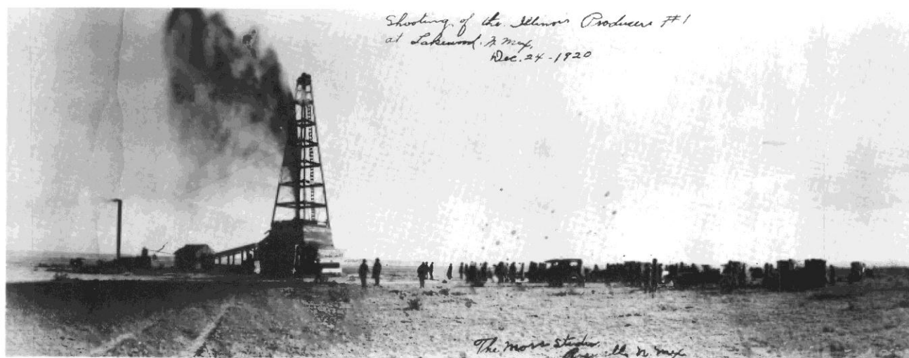
A nitroglycerine charge opens up first producing oil well of the middle Pecos Valley area on December 24, 1920. Photograph by Moss. Courtesy of Southeastern New Mexico Historical Society of Carlsbad.
