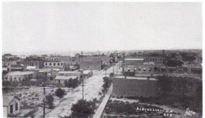
Albuquerque. 1891. July. Gold Ave. - looking east. This photo was probably taken from the San Felipe Hotel (Elk's Club) (5th and Gold). The Central Bank and the Whiting Bldg. can be clearly distinguished in the background (2nd and Gold). Note boardwalk. (U.N.M. Library collection)
