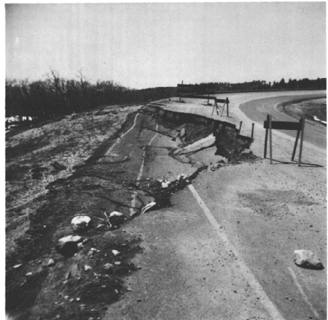
Figure 4. Upper section of the fill-slope failure near Station 643+00. Another failure lies immediately behind the photographer.
