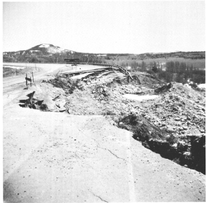
Figure 3. Fill-slope failure at Station 589+50. The hole at the right foreground was caused by erosion through a gap in the severed box culvert.
