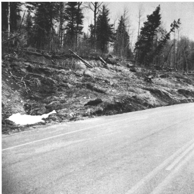
Figure 1. Cut-slope failure near Station 700+00. Note the leaning trees and the scarp where toe material has been removed from the roadway.
