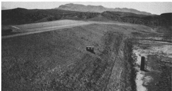
Photo by Soil Conservation Service Figure 1. The Broad Canyon Dam
