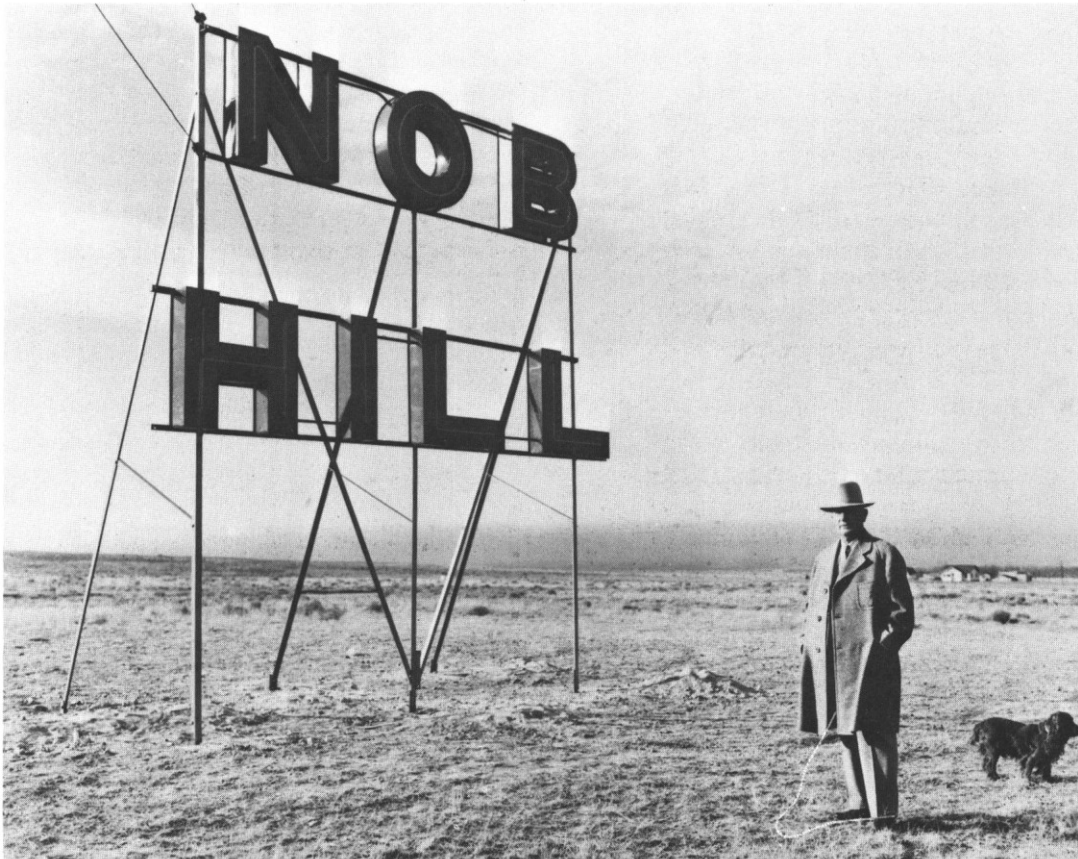
Early construction at Nob Hill. Note early smog in background (Albuquerque Museum Photoarchives).
