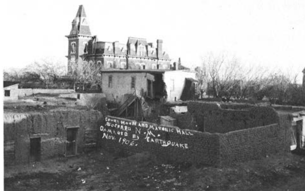
Figure 2. Damage to the old Socorro Courthouse and the Masonic Hall caused by the November 15, 1906 earthquake. Joseph E. Smith photo, November 1906, New Mexico Bureau of Mines and Mineral Resources collection. Courtesy of Edward Smith.
