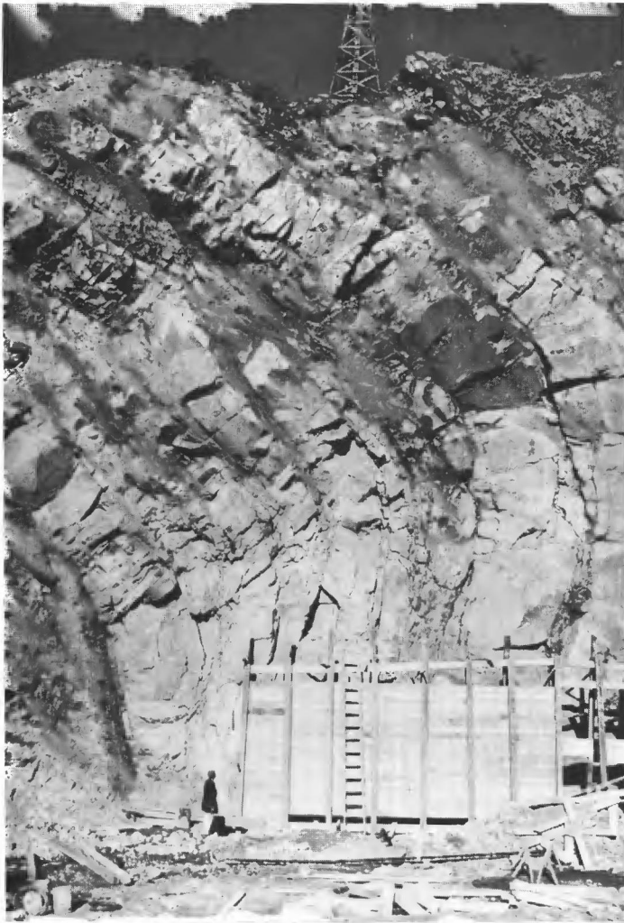
FIGURE 2A-3.8d—Looking west along dam axis at an early stage of construction. Folded and fractured Mesa Verde Gr. sandstones provided less than ideal footing for the dam. Grouting was used to strengthen the bedrock. One version of these events is given by the following quote from the papers of Eldred Harrington: “. . . After the funds had been made legal the site of the dam was changed. So happened that the new site was not a good one, geologically. And yet after all of those years of trials the people in charge wanted, desperately, to build the dam. ‘This is our first chance and if we back down on this one it may take many years for us to get another chance!’ . . . The management called in FAYETTE JONES as a consultant. Jones was the new President of the New Mexico School of Mines. He and JIM FRENCH, an old time civil engineer, looked over the site and cried aloud at its problems. But it had to go on. Jones borrowed a bunch of diamond drilling equipment from the Chino Copper Company just south of Silver City. He riddled the foundation site with diamond drill holes. The crew designed various kinds of pumps, some of them not unlike the familiar ‘plunger’ or ‘plumber’s friend,’ and forced many tons of concrete and sand mortar into those holes. It was quite likely one of the first ‘grouting’ jobs in the world. The grouting job held; it is still holding up well, after more than 60 years.
