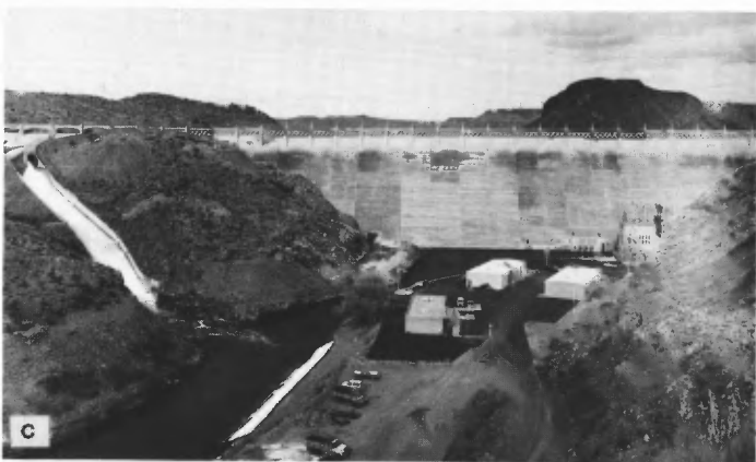
FIGURE 2A-3.8a, b, c—Sequence of photographs illustrates three phases of Elephant Butte Dam construction. (a) 29 May 1912 photograph shows small work area and construction of flume into which the river will be diverted during construction. Towers left and right are part of a cable-transport system that delivered construction supplies to the dam site. (b) Progress of dam construction by 28 October 1914. River has been diverted into flume and the dam is about half finished. At a later stage water was diverted through the powerhouse gates and the flume was blocked by an earthen dam so that the western portion of the dam could be completed. (c) Modern view of dam taken from nearly the same view point on 21 March 1986. Photographs (a) and (b) courtesy U.S. Bureau of Reclamation.
