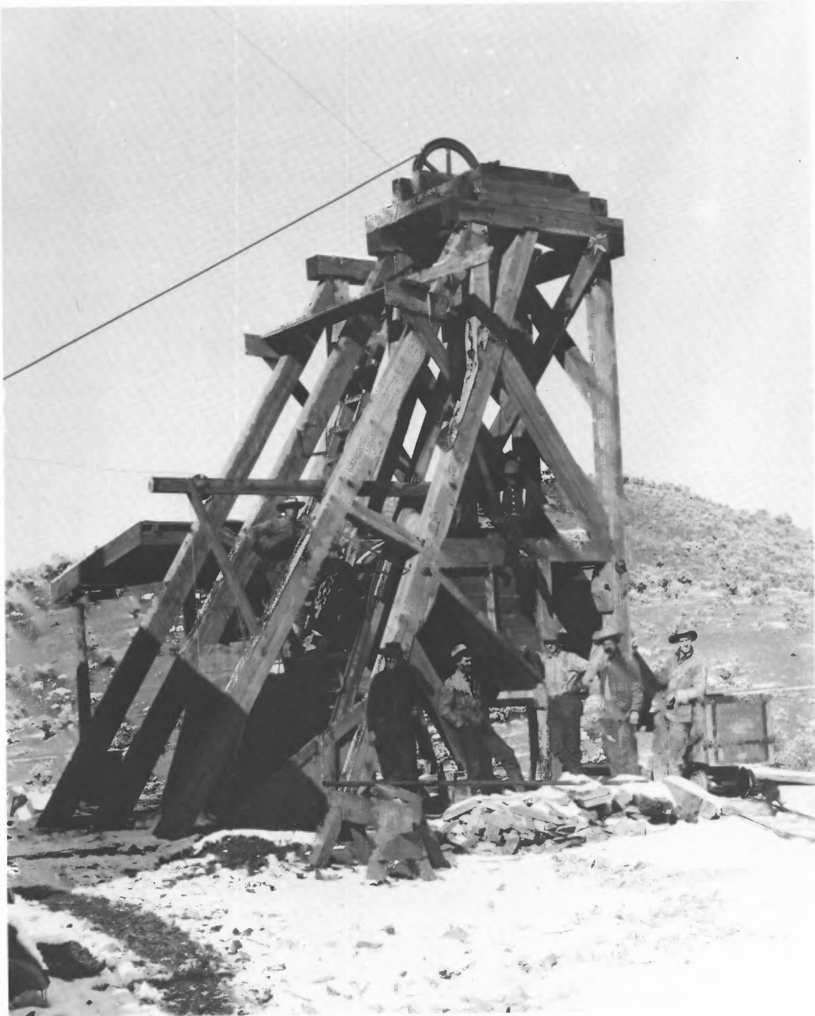
Headframe of U.S. Treasury mine near Chloride, late 1909. Photo Henry Schmidt, New Mexico Bureau of Mines & Mineral Resources Collection, donated by R.H. Jahns.
