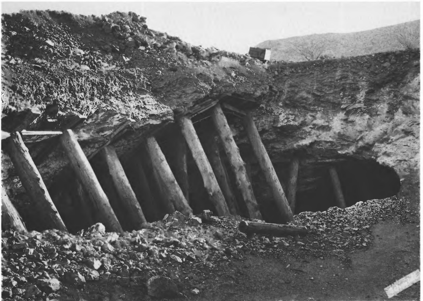
FIGURE 2—Open cut and stope, Carolina claim, Lake Valley, New Mexico, ca 1890. This view has often been identified as the Bridal Chamber itself, when in fact it is more likely the location of Daly’s exploration drift which eventually broke into the Bridal Chamber several hundred feet away. The ore zone has subsequently been stoped out around the original drift, leaving the opening seen here. Photo Henry Schmidt, NM Bureau of Mines & Mineral Resources Collection, courtesy Richard H. Jahns.
