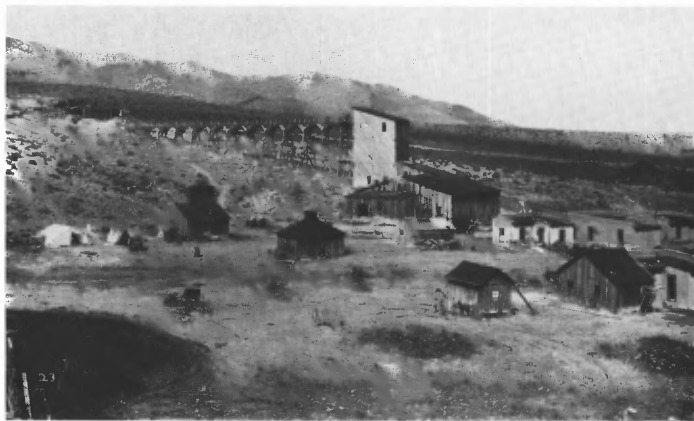
FIGURE 2—Southwestern Lead and Coal Company's 50 ton mill ca 1907. The ore, originally from the Rosa Lee and later from the White Swan, was freighted by team and wagon to the dump point (left center) and then hoisted to the mill over the rail tramway. Originally designed to reduce lead sulfide, the mill was not particularly successful in concentrating vanadinite ores even when redesigned. Photo courtesy Mrs. Lydia Key, Black Range Museum, Hillsboro.
