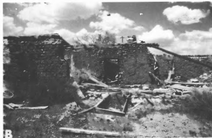
FIGURE 2-106.2a. Abandoned village of Atarque 2 mi west of route at mile 106.2. Photo (A) shows stonework residential building. Photo (B) shows adobe, stonework and stonework plastered with adobe.
