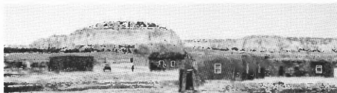
FIGURE 2-106.2b. Atarque as it appeared in 1928. The large structure at right may in part still be standing, and in Figure 106.2a (from Darton, 1928).
