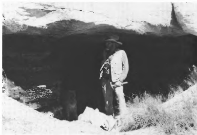
FIGURE 3-54.2. Entrance to School Mine. Coal bed ranges between 4 and 5 ft thick. Note good roof conditions provided by fluvial channel ss. Entrance was sealed and site reclaimed in 1987. Photo by O. J. Anderson in 1982.
