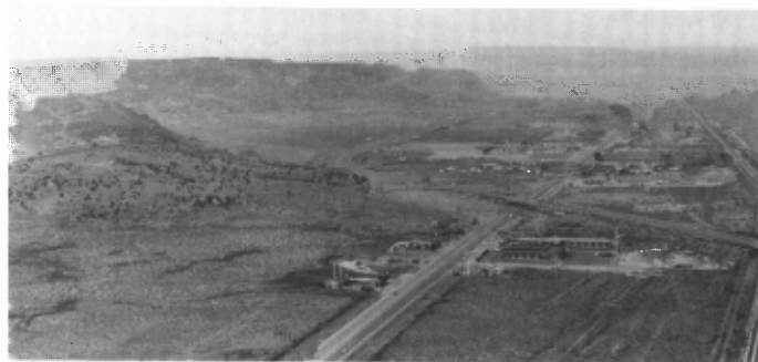
FIGURE 3-0.4a. Aerial view to west from above old US-66. Twin Buttes at left with crushing plant visible, Torrivio anticline is just behind (to the west), identified by the U-shaped notch at center of photo. I-40 overpasses US-66 near right center, and the Santa Fe RR tracks are at far right. Photo by O. J. Anderson.
