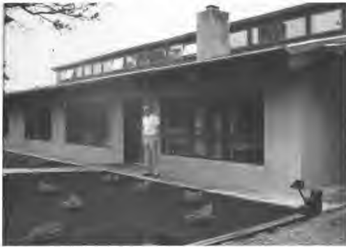
FIGURE 3. Hal Fouts of Gallup, New Mexico, with four untrained helpers produced the walls of his solar adobe home during five months beginning in November 1985 with an Earth Press III machine.
