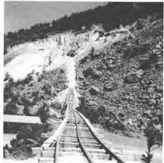
FIGURE 4. Photograph of the pumice operation on East Grants Ridge during the 1940's looking west and upward toward the mine.
