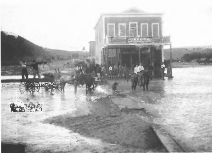
FIGURE 2.2. A late summer freshet has swollen the Cimarron River to the point where the Oxford Hotel is in danger, 13 August 1909. A temporary embankment has been thrown up against the upstream side while a string of planks forms a makeshift bridge. Scenes such as this may have been common along the Cimarron River prior to completion of the Eagle Nest dam in 1918, so common that the photographer seems to be more of a curiosity than the floodwaters. Courtesy Museum of New Mexico. Neg. no. 146899.
