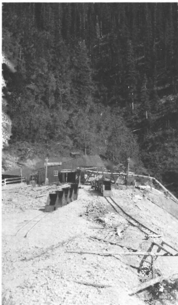
FIGURE 2.17. West portal, Baldy Deep Tunnel mine. At this point the tunnel was 6200 ft in length and the company would soon move to the east portal. From the collection of R. W. Eveleth; photo by Eldred Harrington, 8 August 1926.
