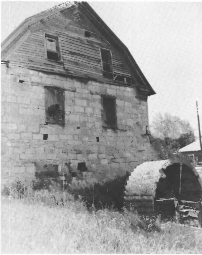
FIGURE 3.12. When Cerain St. Vrain moved from Taos to Mora in about 1885 he bought large tracts of land and proceeded to build a flour mill, several sawmills and even a small distillery. The mill, as shown in this view taken in August 1971, was restored by the county and served as a museum. The Hanosh store in Mora was once the St. Vrain hotel. Photo courtesy of Museum of New Mexico. Neg. no. 53360.
