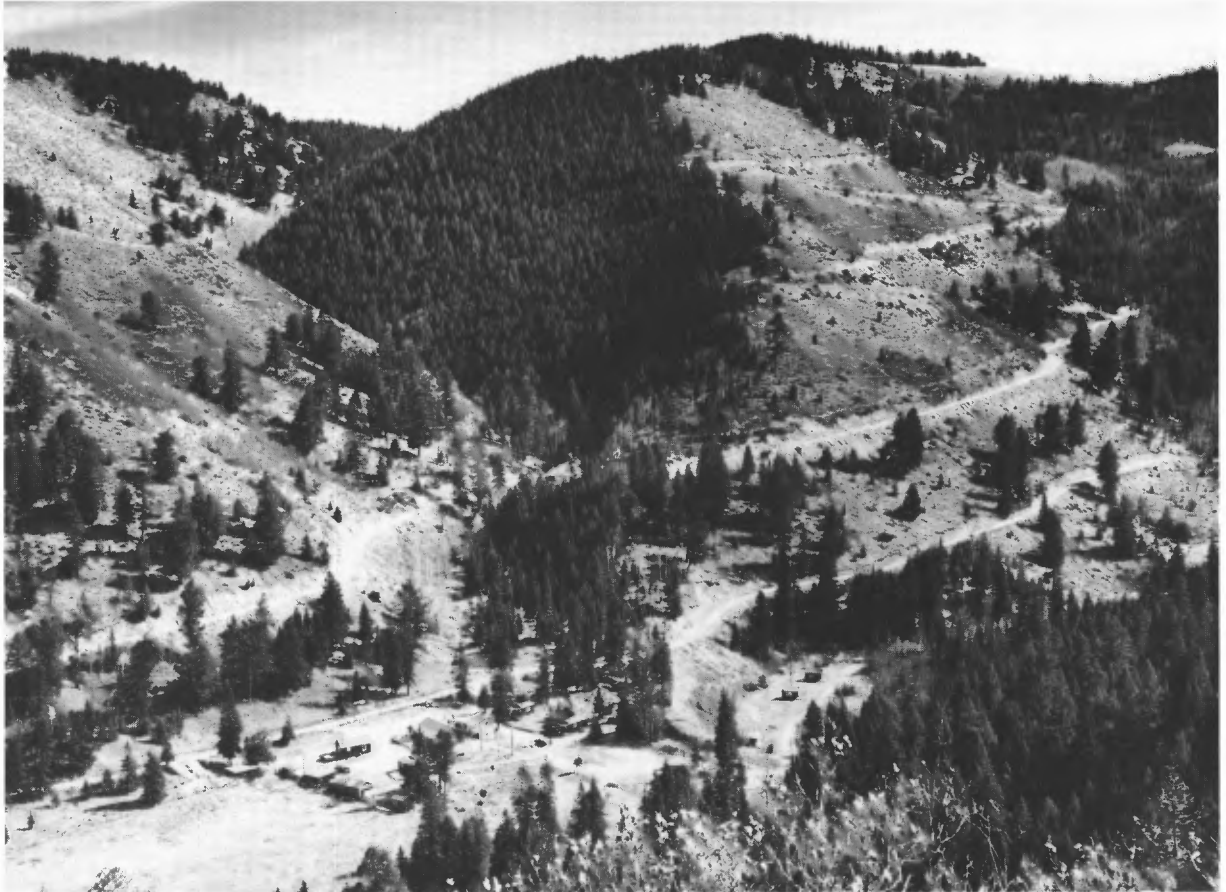
The old Red River Road. This remarkably engineered road was built by the U.S. Forest Service in 1916 to open up the Red River valley to automobile traffic. Prior to 1916, wagons attempting to reach Red River from the east would tie a tree trunk to the back of the wagon before daring a descent down from Red River Pass. The unpaved, single-lane road has a maximum grade of 7.5%, total southern exposure to minimize snow accumulation, makes six switchback turns and climbs 1000 ft. Although this breath-taking road is still accessible, four-wheel-drive vehicles are now required. The new paved road, completed in 1966, follows the canyon of Bobcat Creek to Bobcat Pass, located out of sight to the left. In contrast to the old road, this highway has multiple lanes, steeper grades, fewer magnificent views and is prone to greater snow accumulation. Tall Pines Resort, home of Winifred Hamilton, sits at base of road. The photographer, Harold D. Walter of Santa Fe, was the first person to recognize that Wheeler Peak was the highest spot in the state. Courtesy of Mrs. Winifred Hamilton.
