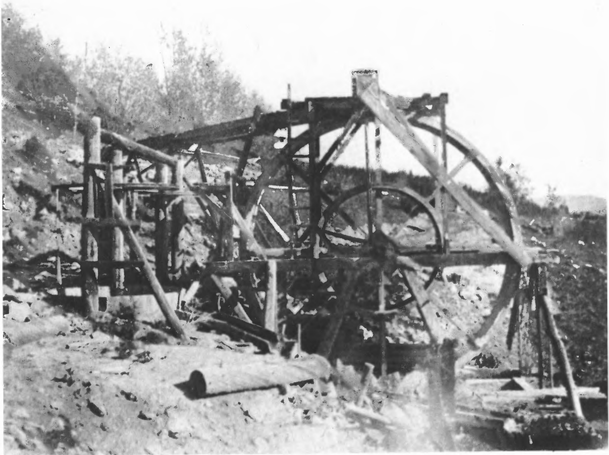
Water wheel built by George L. and M. Read Oldham on the Golden Treasure #1 claim in Placer Creek, Red River District, circa 1898. A 2-mi ditch was built to carry water from Goose Creek to this wooden wheel and arrastra (crude mill located to left of wheel) on the East Fork of Placer Creek. Mine shafts on the Golden Treasure were plagued by excessive water, and gold production was unimpressive. As a testimonial to the superb craftsmanship of the Oldham brothers, the 92-year-old water wheel on Placer Creek still stands. This is one of three water wheels said to have operated in the Red River area near the turn of the century. Courtesy of Mrs. Winifred Oldham Hamilton.
