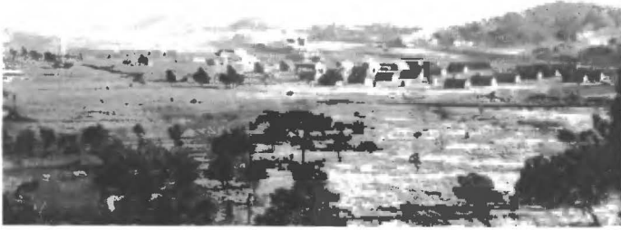
FIGURE 3.13. The coal mining camp at Coalora, New Mexico, around the year 1900 (Photo courtesy of Mr. J. N. McDaniel, Carrizozo, New Mexico).
