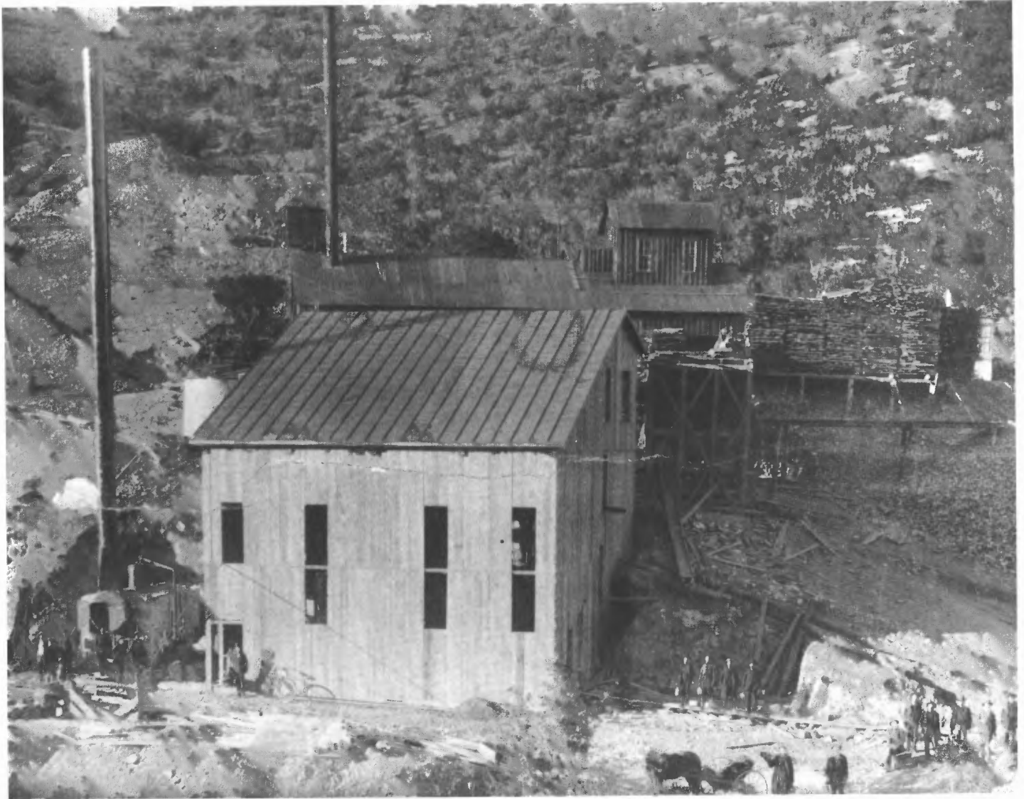
The Old Abe mill, northwest of White Oaks, had just been completed when C. W. Marks made this view in circa 1893. The Old Abe shaft is hidden in the structure behind the mill. Note that the boiler is not yet closed in from the elements and windows are yet to be installed on the mill building. At least one person preferred the bicycle to the horse when traversing the two miles between the Old Abe and White Oaks. New Mexico Bureau of Mines collection No. 1666, courtesy of Dr. Richard H. Jahns and John Kelt.
