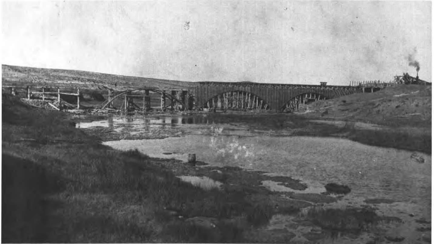
FIGURE 3.19. Construction begins on the concrete flume over the Pecos River near Carlsbad Springs (January 16, 1903). The earlier wooden flume (constructed 1889–90) at this site was ruptured numerous times by floods starting in 1893. Type Tansill area and Ocotillo Hills are beyond the flume on the west side of the river. Courtesy of Southeastern New Mexico Historical Society of Carlsbad.
