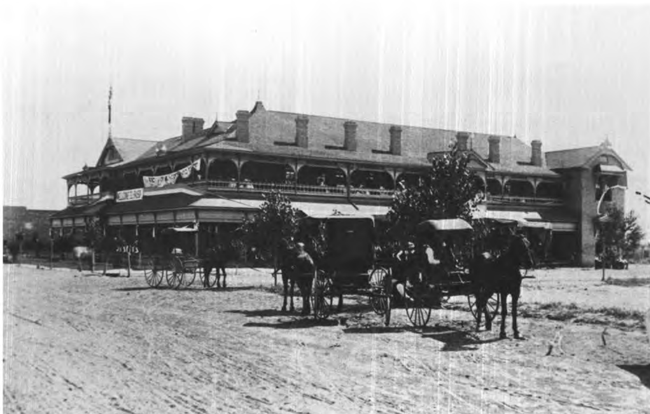
FIGURE 3.20. Little Eddy had a surprisingly large hotel. It was built by the Town Company to convince potential land buyers that Eddy, New Mexico, was here to stay. Photograph by Stringfellow, January 4, 1891 (neg. 14605), courtesy of Museum of New Mexico Collections.
