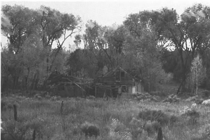
FIGURE 2.14. Ruins at Gabaldon homestead.
