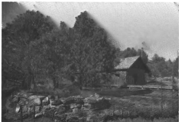
FIGURE 2.7. View north, across NM-223, of the well and adobe remains of Pigeon's Ranch, a major Santa Fe Trail way-station. The original 23-room complex was built by Alexander Valle in the 1850s. The ranch was prominent in the Battle of Glorieta, serving as a field hospital and morgue.
