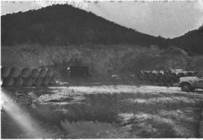
FIGURE 3.16. Carache Canyon exploration decline and stacks of ventilation ductwork.
