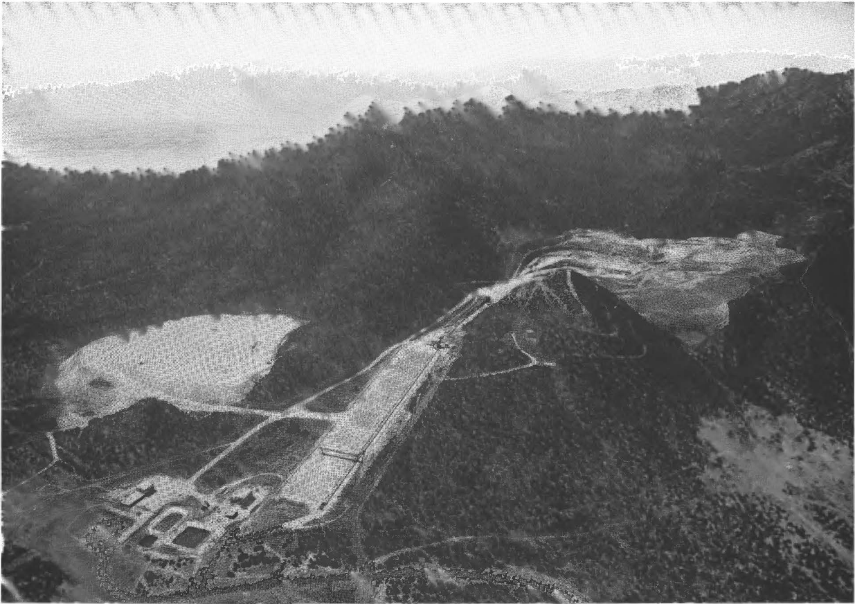
FIGURE 3.14. Aerial view of Gold Fields Cunningham Hill mill and mine in early 1980s. Photography and flying by Paul Logsdon.
