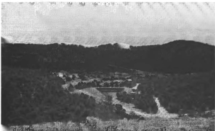
FIGURE 3.15. Acid drainage catchment pond at base of reclaimed and revegetated mine waste pile in Dolores Canyon. View north from top of mine waste pile.
