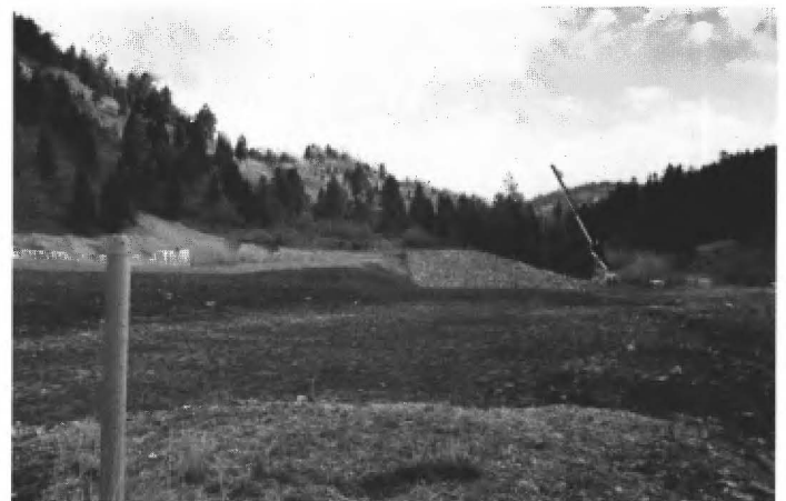
FIGURE 2.21. View looking north up the Redondo Creek graben from the former site of the Baca-6 well (marked by the pole). The gravel embankment and concrete retaining wall were to protect the proposed 50 MW(e) geothermal power plant that was never built on this prepared pad. Arrow points to a group of people for scale.
