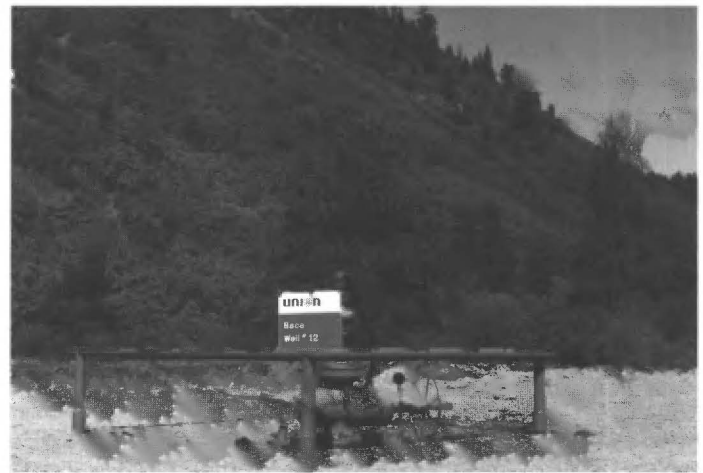
FIGURE 2.16. Wellhead of Baca Well #12, the deepest and hottest well drilled in Valles caldera. Intracaldera Bandelier Tuff is exposed (in background) in the walls of Redondo Creek graben.
