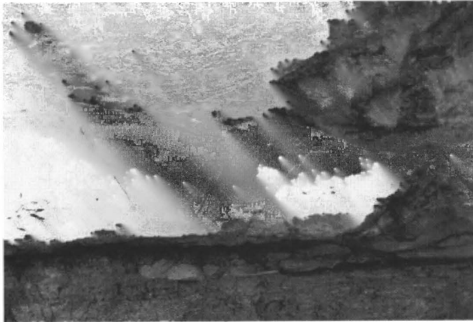
FIGURE 7: Conjugate shear joints observed in Point Lookout Sandstone. Ledge-forming sandstone unit is approximately 1ft thick.
