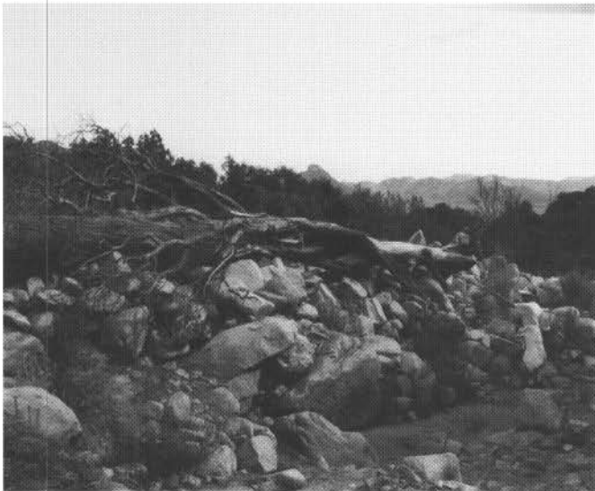
FIGURE 11. Marginal rock levee along the west bank of the lower active channel of Anvil Creek, approximately midway between the breach and the loop road. Although the large tree was rafted a considerable distance, its bark and branches survived mostly intact.
