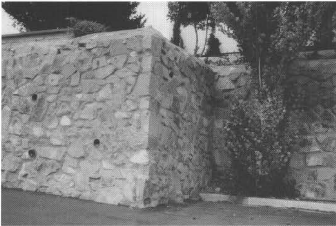
FIGURE 4. A stone wall constructed of concrete and Vado Andesite in Las Cruces.
