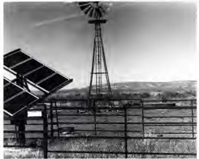
FIGURE 2.3. Solar-powered well at mile 28.2.
