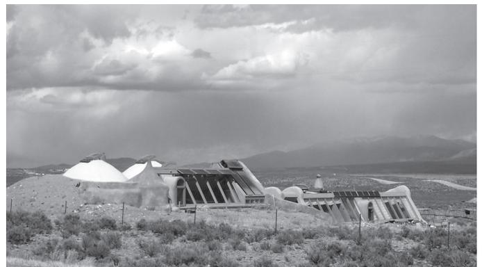
FIGURE 1.24. Earthship homes were popularized by actor Dennis Weaver, whose beautiful and efficient home in Ridgway, Colorado incorporated used tires, aluminum cans, and other recycled materials in its structure. Earthships, such as this Taos County home, are passive solar designs that use thermal mass to regulate seasonal heating and cooling requirements. Electricity is supplied by photovoltaic panels.
