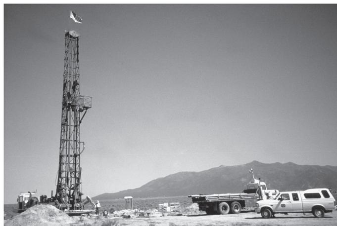
FIGURE 2.18. Photograph of the August 2001 drilling of the 2039-ft-deep BOR-6 production well 4 km northwest of STOP 2. This was one of six deep wells that were drilled around 2001-2 in order to provide hydrogeologic and hydrologic data to support the water rights settlement for the Taos valley. Surprisingly, the well encountered Servilleta Basalt at over 1000 ft depth, suggesting that either Pliocene basalt flows filled a deep valley, or the basalt is downfaulted.
