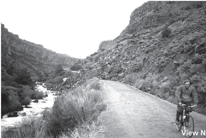
FIGURE 2.37. View east along the Rio Pueblo de Taos of the 57,000-ton landslide that blocked NM-570 on February 3, 1993. The slide is developed in Pleistocene landslide deposits of Servilleta Basalt and interlayered sediment. The breakaway zone is well-defined, and visible in upper right corner of photo. Original road construction removed the toe of the naturally oversteepened slope, creating a wide zone of unstable material.
