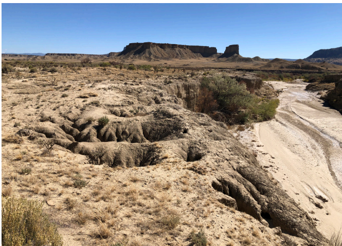
FIGURE 2.61. Piping features on the north side of the recently incised wash of Arroyo Chico. View to east. Butte in background is capped by the Dalton-Hosta sandstone tongue, which overlies the Mulatto Tongue of the Mancos Shale.
