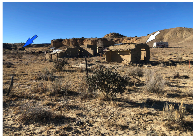
FIGURE 2.65. View to west-southwest of three abandoned adobe structures in Guadalupe. A modern residence lies behind, near the foot of the bluffs capped by Gallup Sandstone. The blue arrow denotes the location of Ojo de Padre spring, which likely discharges from a sandstone bed in the uppermost part of the lower tongue of the Mancos Shale. The white arrow points to the Catholic church. Adobe buildings behind and to the left of the church probably included the school and dancehall (per fig. 1 of García, 1994).
