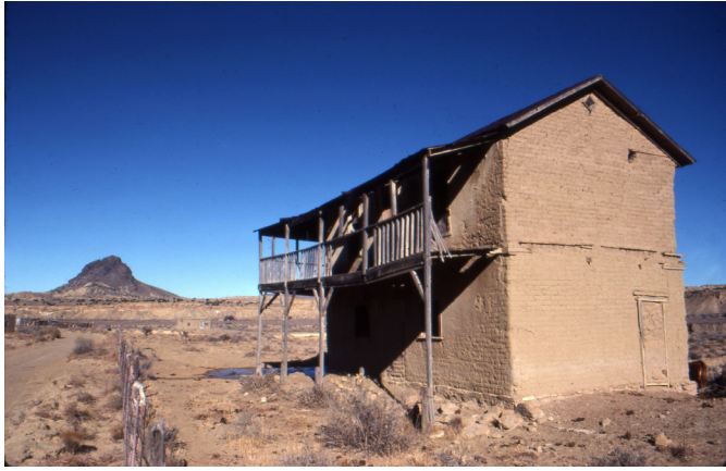
FIGURE 2.66. Juan Córdova store and residence (lower and upper stories, respectively), as it looked in 1981.
