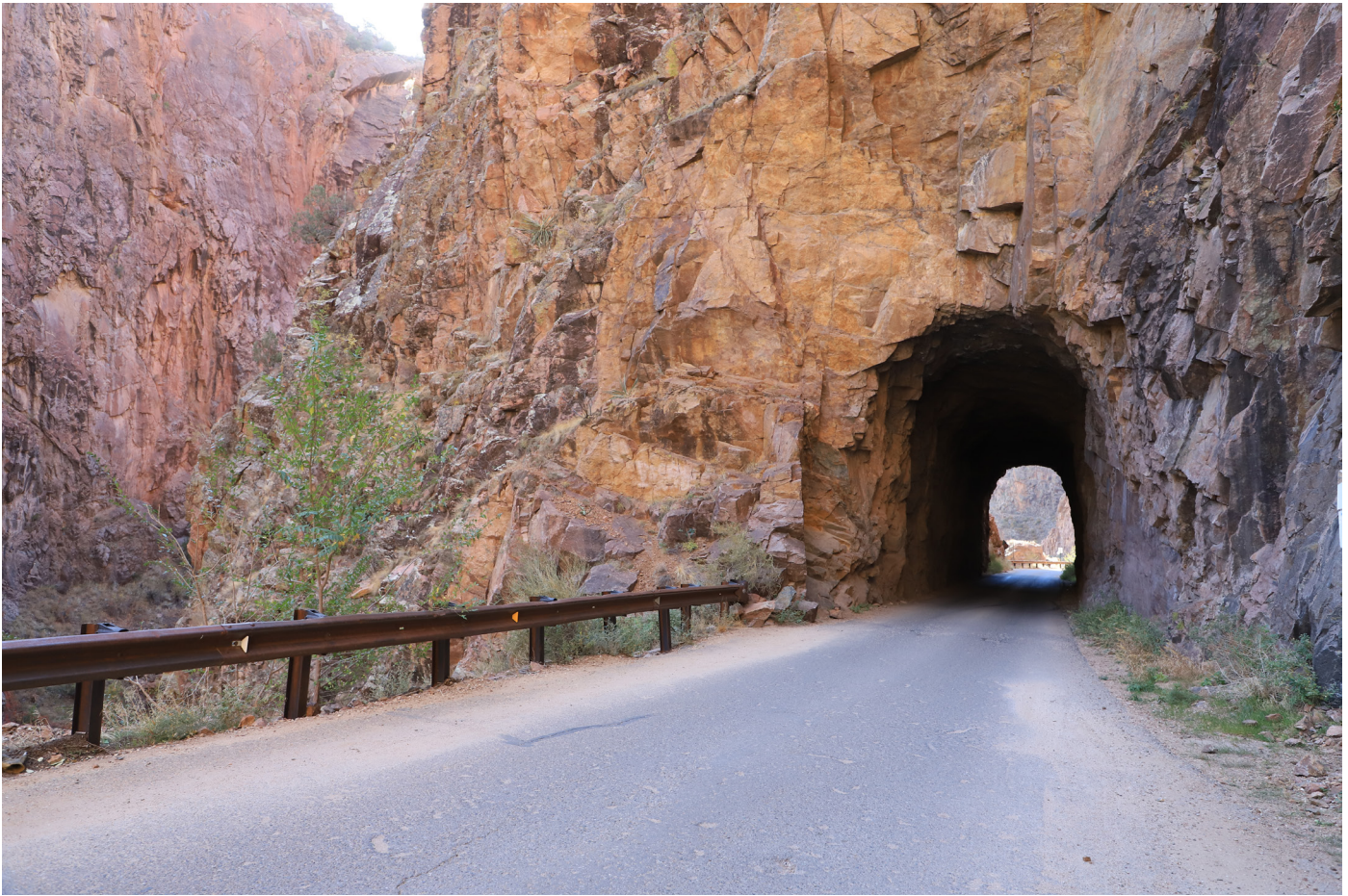
FIGURE 3.6. Gilman Tunnels were cut through Mesoproterozoic granite and have a very tall profile to allow the passage of narrow-gauge trains carrying logs from the Nacimiento Mountains to a sawmill in Bernalillo from the 1920s to 1941.
