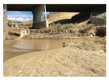
Figure 1.65. Photograph of engineered stone steps installed in 2005 beneath the lower U.S. Route 550 bridge over the Rio Puerco. View is toward the east (upstream). Note erosion on right side of photo. Taken from Loberger et al. (2021).
