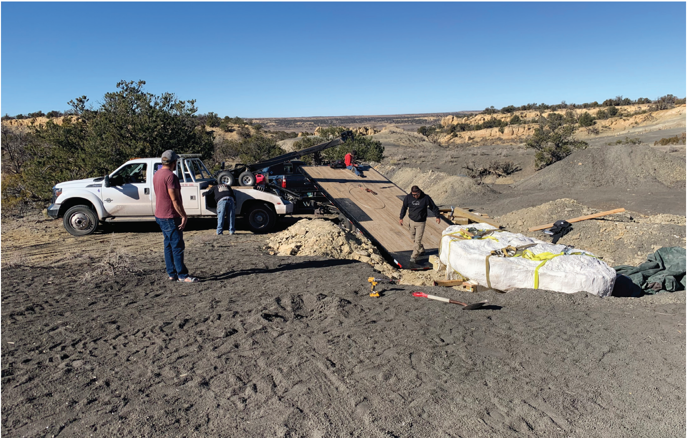
Figure 10. Car hauler trailer tilting bed under the skis of the sled.
