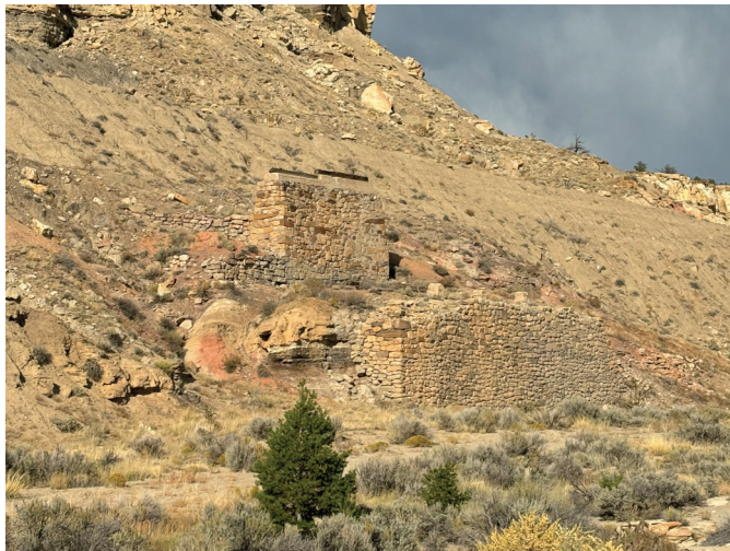
Figure 2. Historical (top) and modern (bottom) photographs of the tipple at the San Juan mine (location in Fig. 1). View is to NNE. The lower rock wall of the tipple foundation is an estimated 5–6 m (~15–20 ft) tall. Historical photograph taken by W.G. Pierce (per Dane, 1936).
