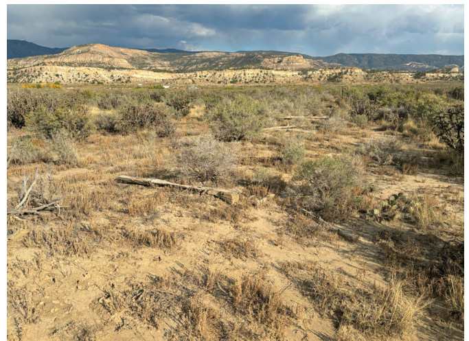
Figure 4. Photograph of the railroad spur leading to the coal tipple, with some wooden ties remaining. The earthen foundation (bed) of the railroad is raised about 0.5 m (1.5–2 ft) and no gravel was used.
